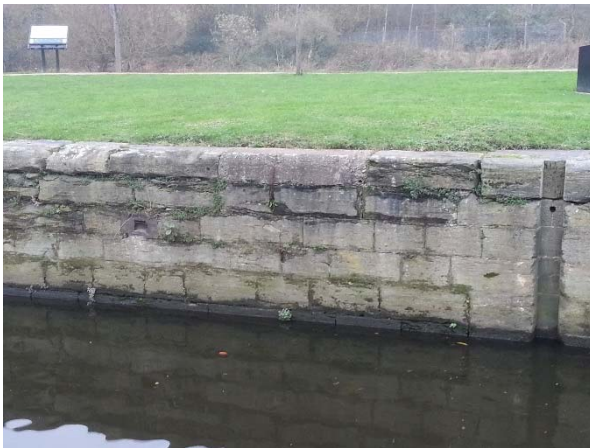
Photo 7: Typical material along Knothrop Cut
