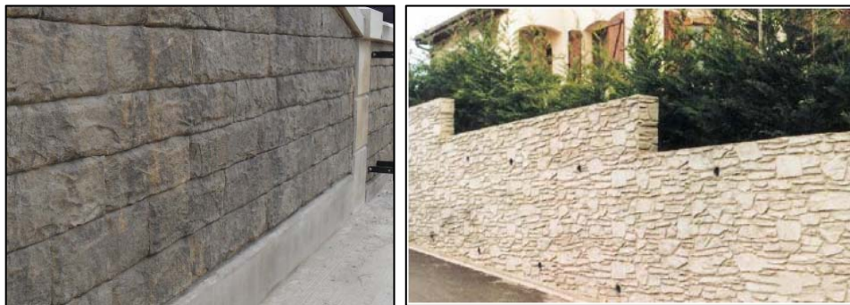
Photos 10 and 11: Pigmented Concrete with masonry imprint
