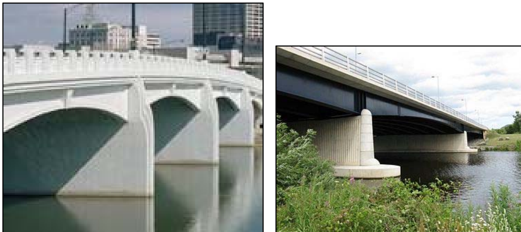
Photos 12, 13, 14 and 15: High Quality Concrete finishes on bridge piers
